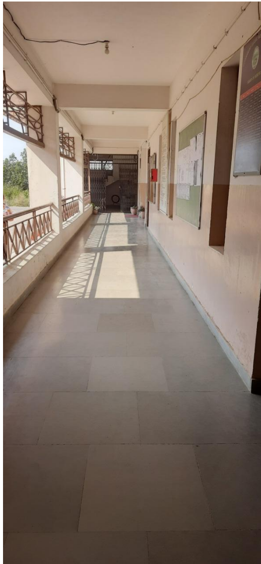
Cleanliness in Building
