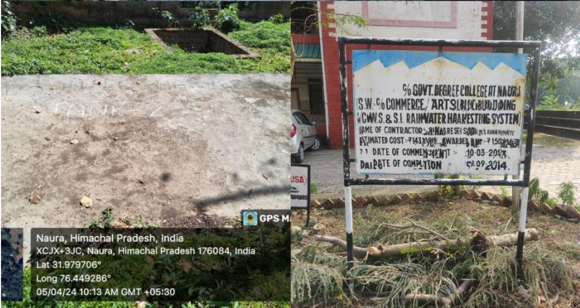
Rain-Water harvesting tank
